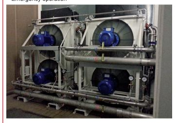
AC-MS Compact - Modular table coolers Cooling systems for gas compressor power station
