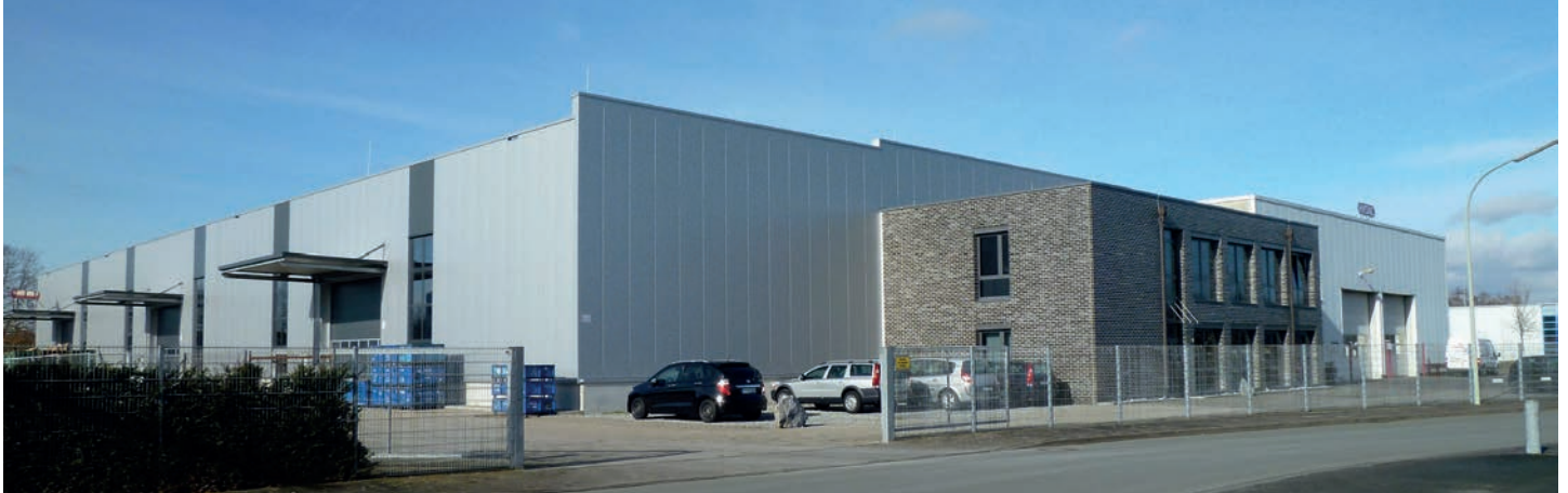
Plant HYDAC Accessories - Servicestelle Nord, Rheda-Wiedenbrück
