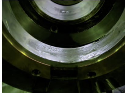
Fig. 1: Damage of sealing surfaces
