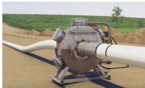
▪ step 2: crimping of sleeve
